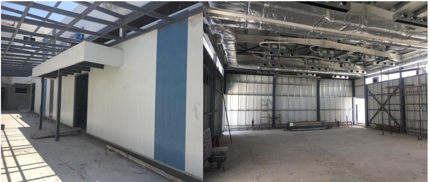
Figure 5: Two new classrooms under construction (total area: 220 m 2 – total capacity: 140 people).
